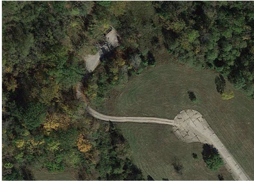
Figure 3-21: Ethans Glen WWTP
