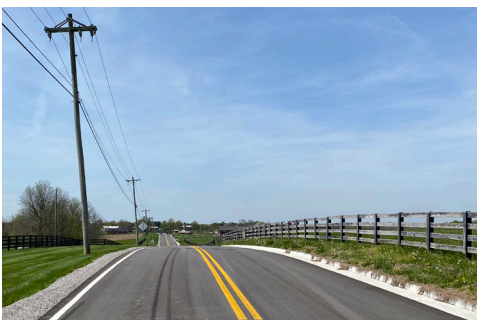
Porter Road near Walton-Verona Elementary School. Recent upgrades improved safety and access while preserving the rural character.
