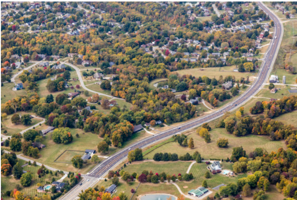
The Pleasant Valley Road (KY 237) corridor with Valley View Drive near the bottom of the photo.
