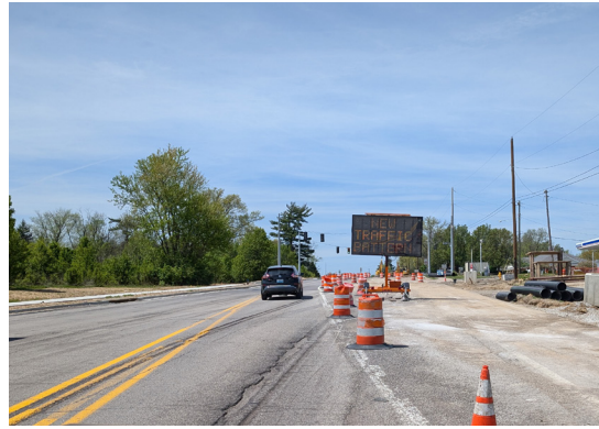
A message board sign on Donaldson Highway at the Boone/Kenton County line warns drivers of a new traffic pattern due to ongoing construction of a transportation improvement project.
