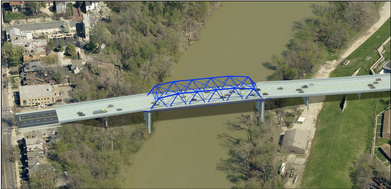
Figure 24: Truss Alternative Layout
